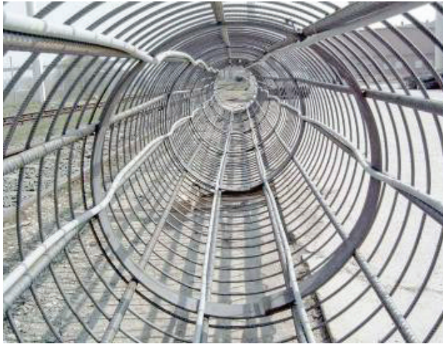
PEX in rebar cage/structural pile
