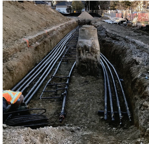
HDPE buried headers
